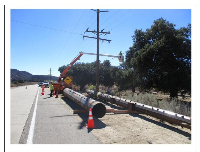
**Photo 4:** A construction crew observed trimming a nearby oak at Z40539 (TL 629C) for pole installation and line clearance.
