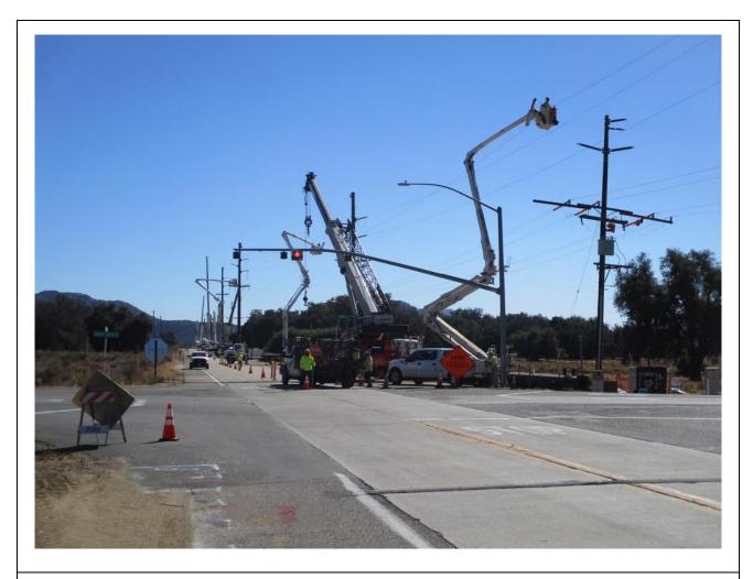
**Photo 6:** A construction crew observed conducting a lane closure along Old Highway 80 between Z40529 and Z100056 (TL 629C) and using a pilot car to lead motorists around construction areas in accordance with APM TRANS-02.
