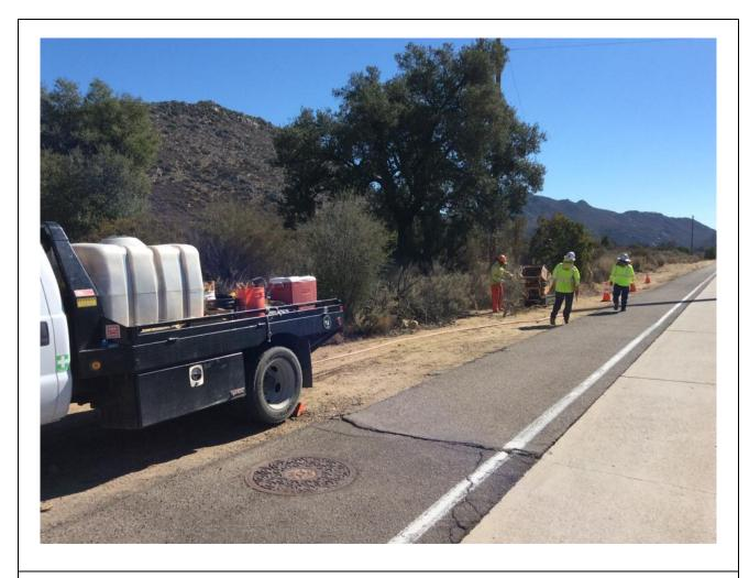
**Photo 5:** During vegetation chipping at Pole Z206014S (TL 629C), the crew was equipped with at least 100 gallons of water with a pump and hose, as required by the CFPPP Fire Matrix for the activity, location, and FPI.
