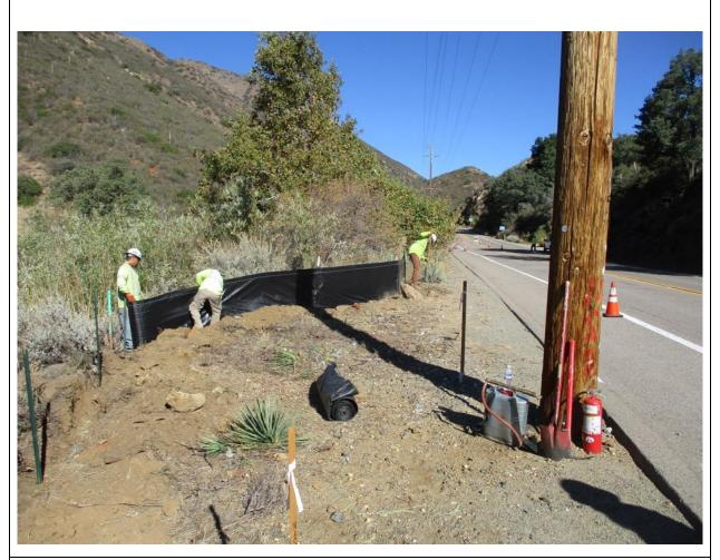
**Photo 3:** A construction crew observed installing silt fence at Z40506 (TL 629C) in accordance with the Erosion Control Plan and SWPPP (MM HYD-1, MM BIO-7) .
