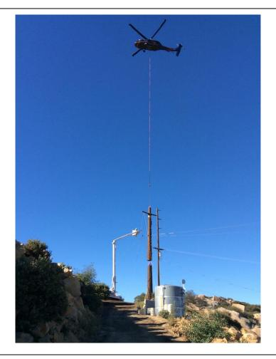
**Photo 1:** A CPUC ECM observed installation of the middle segment of Pole Z571428 (TL 6957) using a helicopter.
